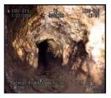
For regulatory reporting, silt, fat, roots debris are all classed as a blockage. However, it is important that the actual cause of the blockage is recorded within the incident record. The response to each of these might require a different solution. For example, a persistent fat problem may require trade effluent control or persistent siltation problems may need to be added to the de-siltation programme for that area.
