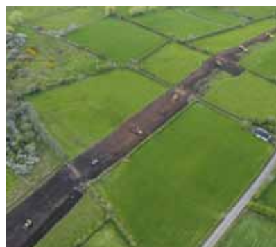
Preparation of the working width.
