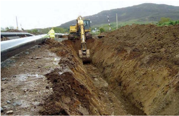
Pipe Stringing and Bending
