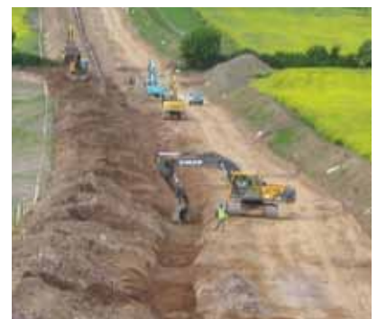
Backfilling.
