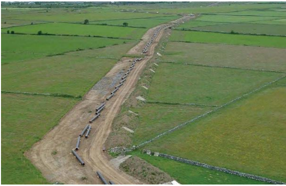
Pipe Stringing and Bending
