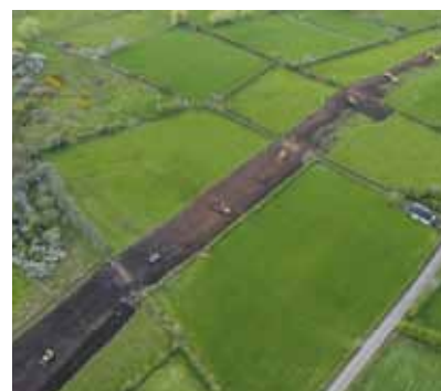
Preparation of the working width.
