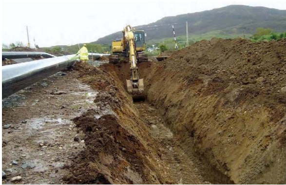
Pipe Stringing and Bending
