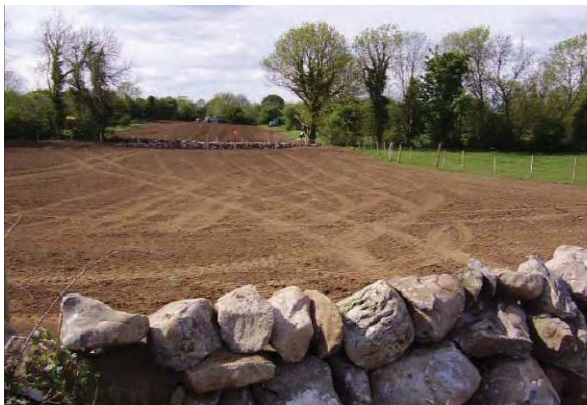
Reinstatement of the Pipeline Spread
