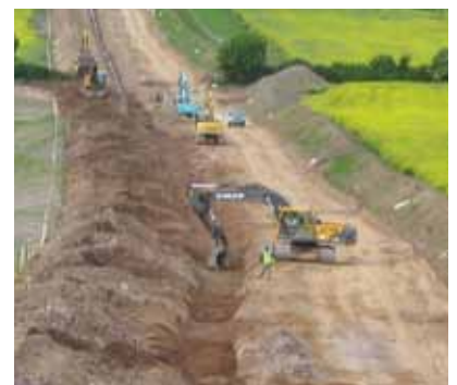
Backfilling.
