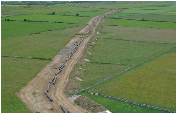
Pipe Stringing and Bending
