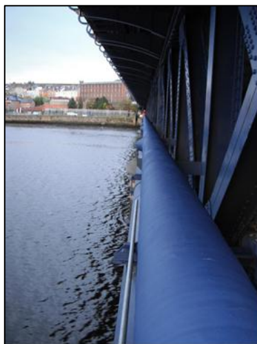
Figure 11.5c: Completed works on the Craigavon Bridge
