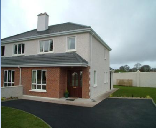
Typical Existing Semi-Detached 100m 2
