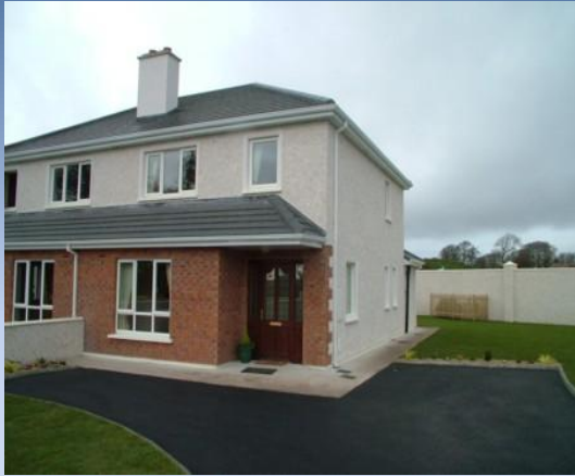
Typical Existing Semi-Detached 100m 2
